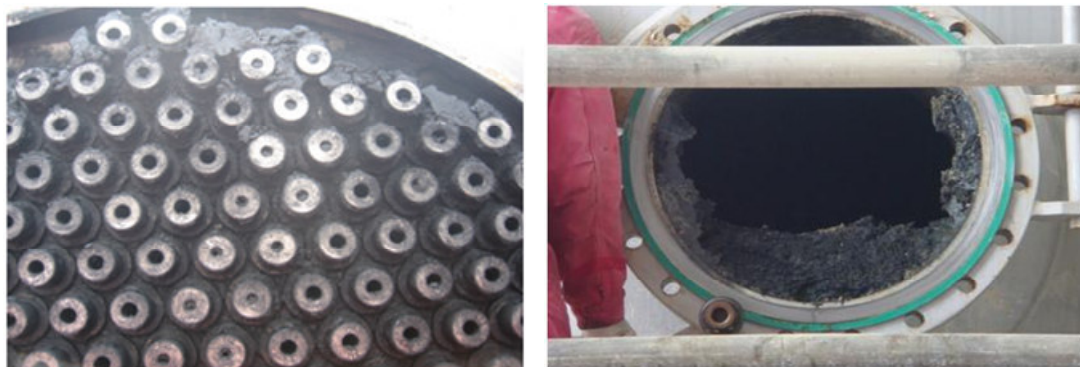
Figure 1. Field A facility. Images showing hydrocyclone package liners and separator coated with CaN solid deposits.
